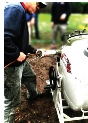
CAMERA INSPECTION PORT
